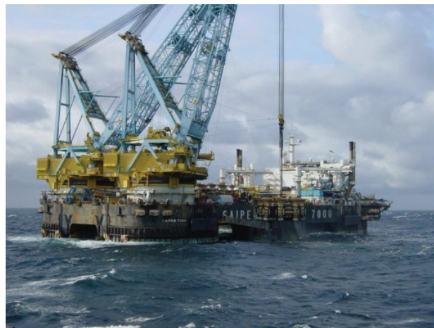
Figure 1 - Hutton Foundation Template Lift-Off from Sea Bed
