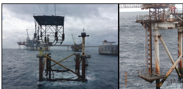
Figure 11- Access Platform to the 2/4S Jacket and Tripod
