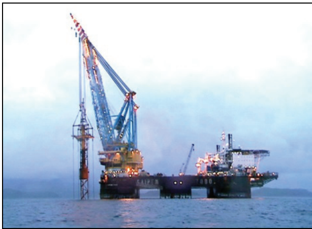
Figure 2 - Brent Flare Tower Lift-Off from Sea Bed
