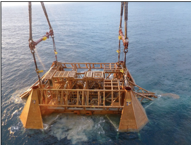
Figure 6 - TOGI Template Lift-Off Near Shore
