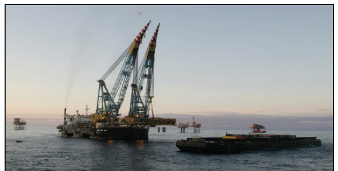
Figure 5 - The 9000t MSF Removal
