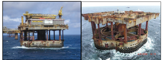
Figure 4 - Concrete Drilling Platform 1 - Platform Before and After Removal
