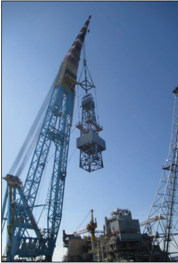
Figure 8 - The Removal of Heimdal Drilling Derrick The second part, including the substructure and skid base, weighed approximately 1000t. Again, the condition and weight data were somewhat vague.
