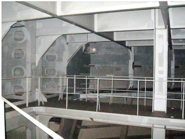
Photograph 1. Ballast tank with well prepared PMA.
