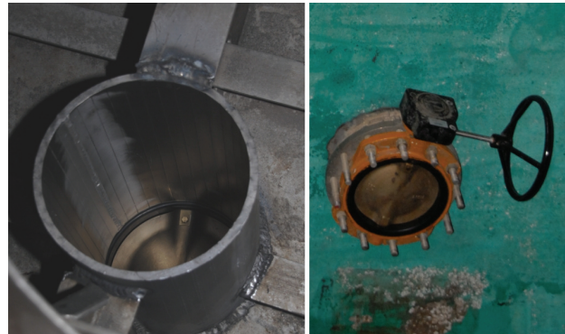
Figure 2: Butterfly valve used as a damage hole
