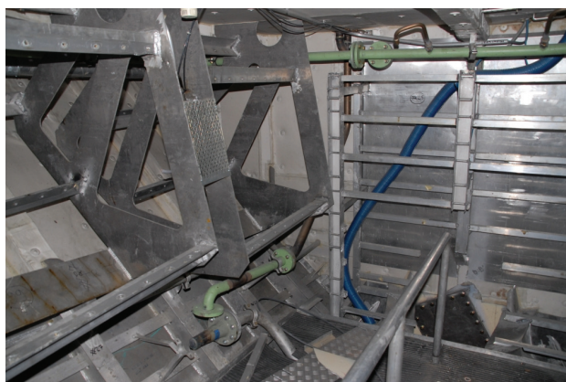
Figure 9: Empty store in the forward compartment
