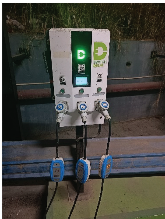
Figure 3. Charging point at Kalkaji Mandir Metro Station
