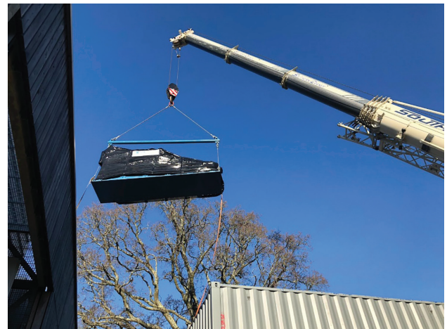
Figure 3. East winch delivery
