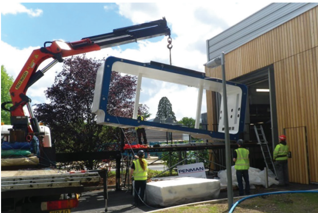
Figure 8. Delivery of a carriage section
