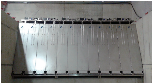
Figure 10. View of the wavemaker after installation
