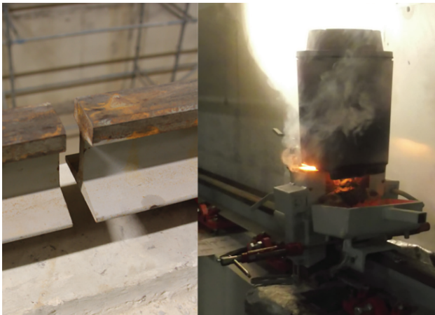
Figure 4. Rail welding
