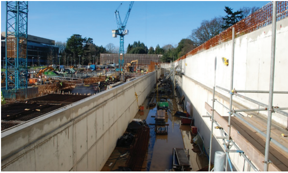
Figure 1. Construction site in February 2014. View towards the West end where the tank had to be cut deepest into the ground
